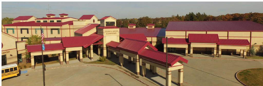
Council Grove Elementary - Oklahoma City, OK
